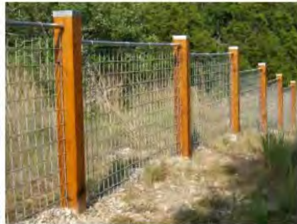
Security perimeter fence (wood post with galvanized wire to prevent corrosion)
