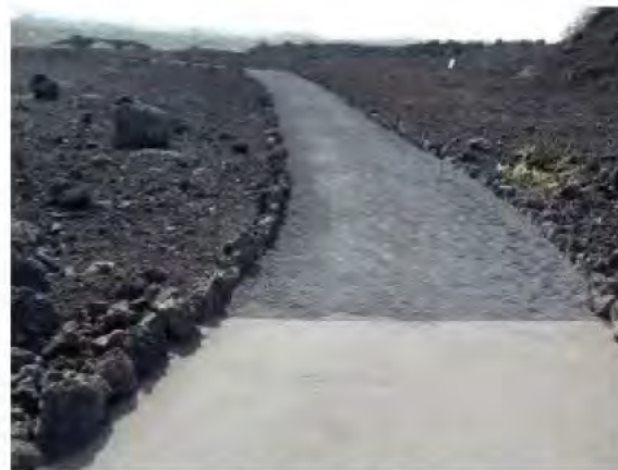
Combination concrete and crushed basalt stone with stone header
