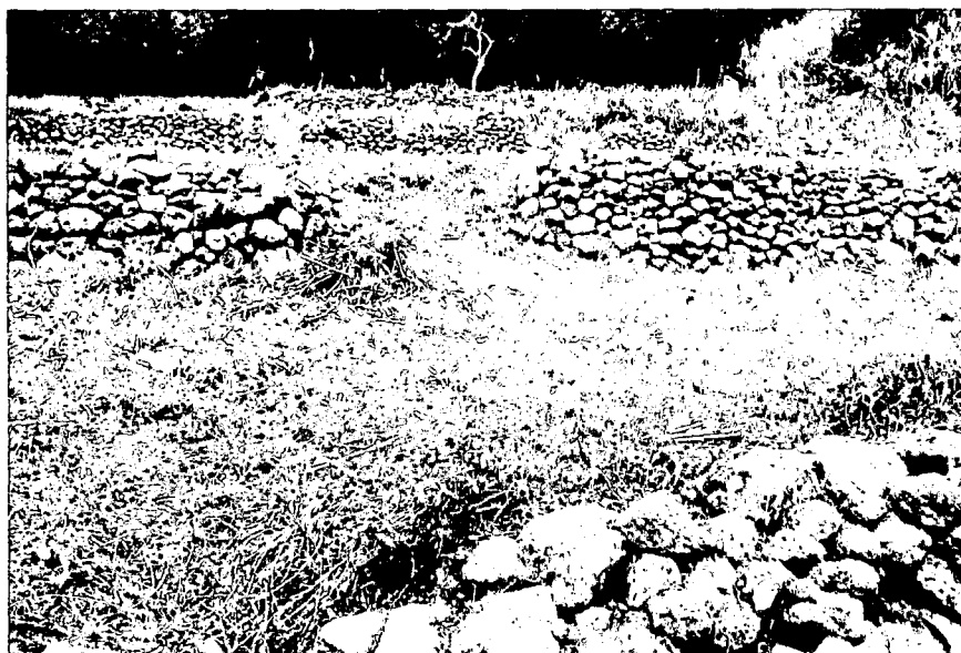
Figure 4-5. Terrace Walls Requiring Repair
