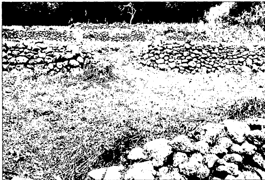
Figure 4-5. Terrace Walls Requiring Repair
