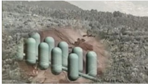
Vertical fuel tanks at Red Hill fuel storage facility. Tanks 1 & 2 are to the bottom right.
