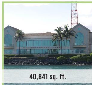
D - 45 Ahui St. and 53 Ahui St.
