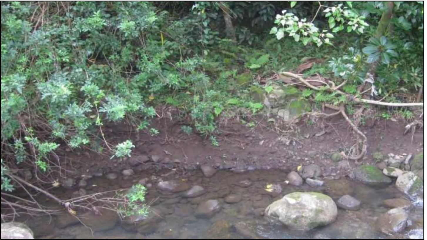
Figure 14 . Edge of Area 6 eroding away from stream wash.
