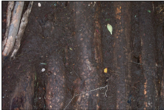
Figure 12. Corduroy is widely used in wet locations as a replacement for costly aggregate, where anaerobic conditions prevent wood decay. It also allows the community to participate in building the road or trail. These examples are from Mexico (top left) and Volcano (top right, bottom right). The initial log layout is bound by either soil or sand to provide a smooth wear surface.
