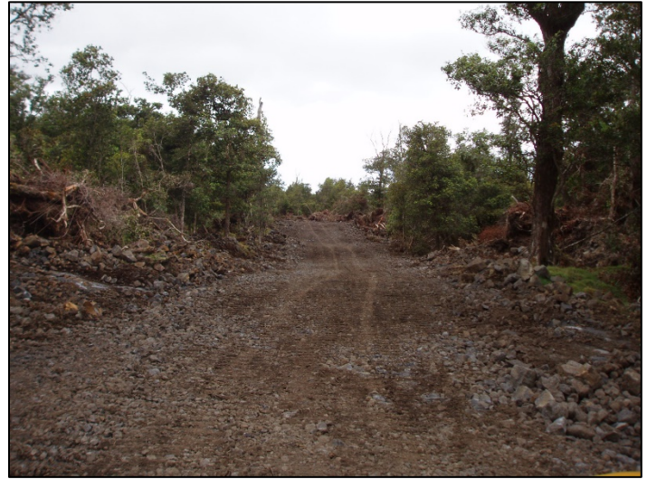
Figure 9. Road alignment should be follow well-drained, stable soil. In Wao Kele o Puna this means staying on recent, more elevated lava flows. In this road, most of the base material is derived on site with considerable savings.
