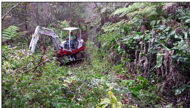
Figure 11. Mini-excavators, now widely available, are a good choice for trail development if manual options are not viable or not available. They can easily move around sensitive areas and do not cause extensive collateral damage. For Wao Kele o Puna, the use of steel tracks will be necessary due to rocky soils.
