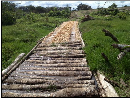
Figure 12. Corduroy is widely used in wet locations as a replacement for costly aggregate, where anaerobic conditions prevent wood decay. It also allows the community to participate in building the road or trail. These examples are from Mexico (top left) and Volcano (top right, bottom right). The initial log layout is bound by either soil or sand to provide a smooth wear surface.
