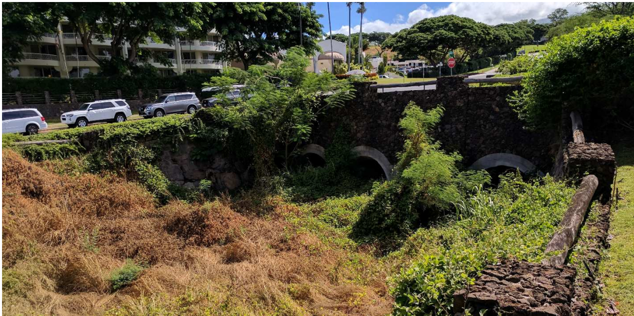
Photo 7: Looking upstream toward the four 90" drain lines crossing under Ualei Place
