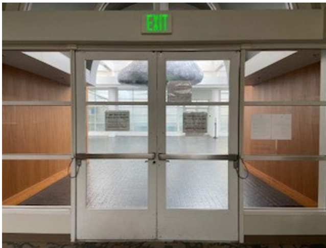
Figure 2 – View of the Double Doors Inside the BOT Office
